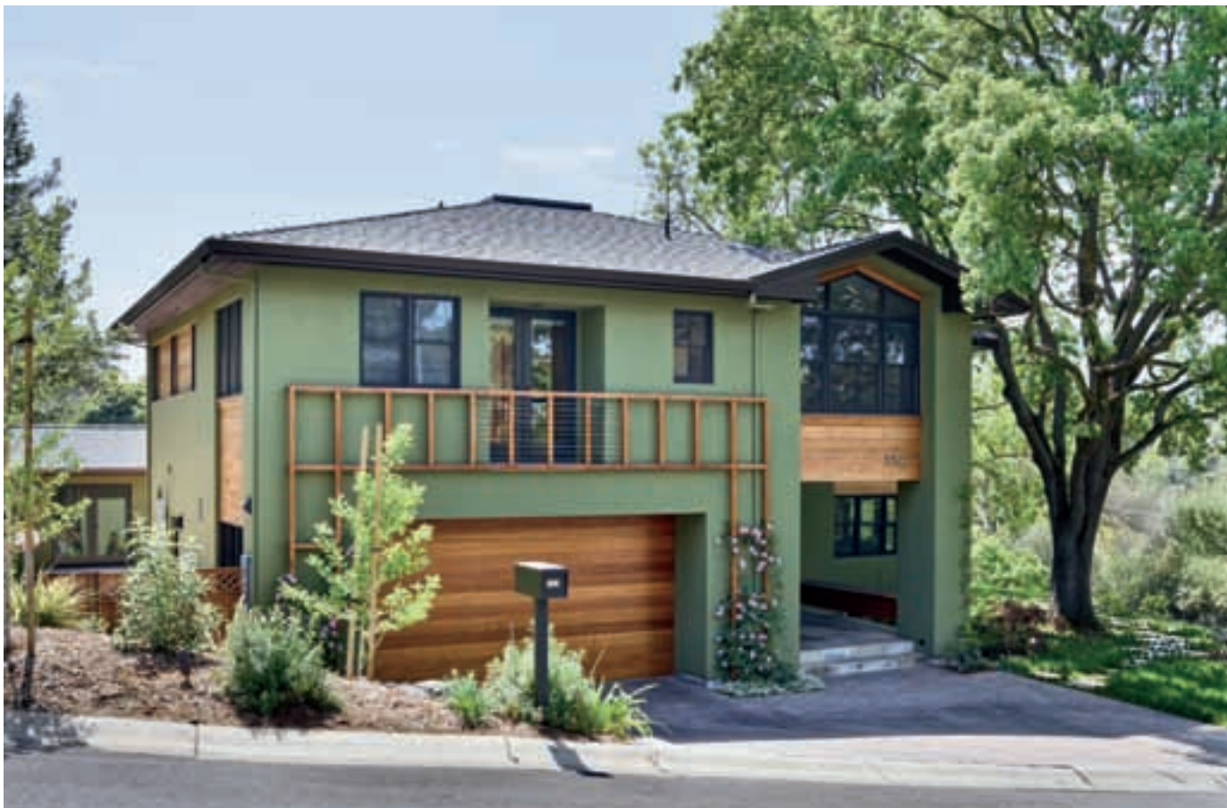
Figure 14: Documentary architectural photograph
